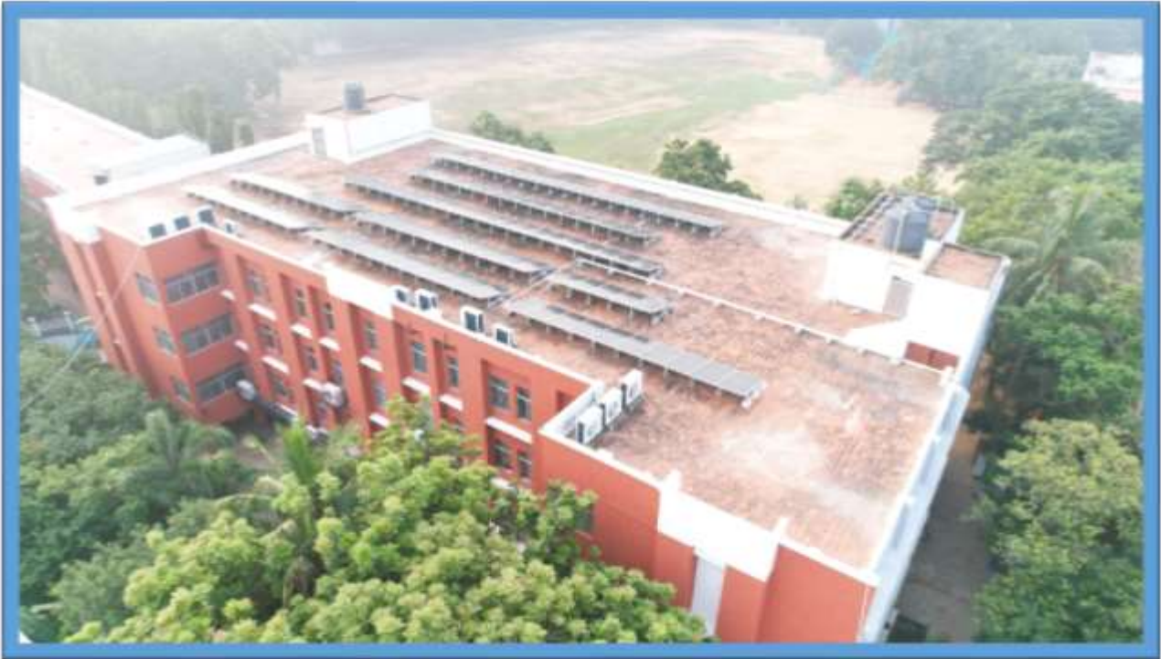
D Block Solar Panels
