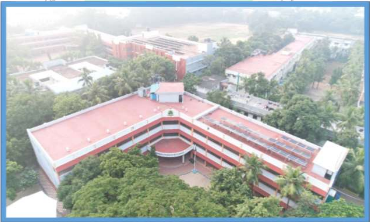
Aerial View of Solar Panels
